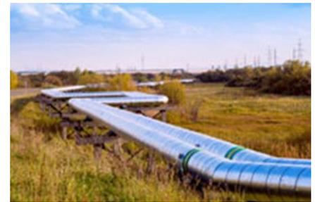
*This hot-water pipeline appears to be fine during visual inspections. As we will mention later, there are many thermal bridges on this pipeline that reduce the efficiency of the transport of thermal energy. Traditional cameras do not detect defects on internal heat insulation and leaks below the surface of the ground.*
