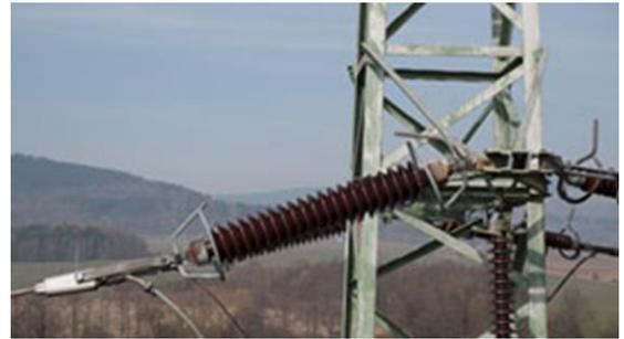
*Photographic image from an aviation inspection of high-voltage distribution lines. Although there is nothing to be seen on the photo, there is a defect on the joint in the form of high transient resistance. The electric joint has become overheated and according to the recommendation in ISO 18434-1 should be repaired as soon as possible.*
